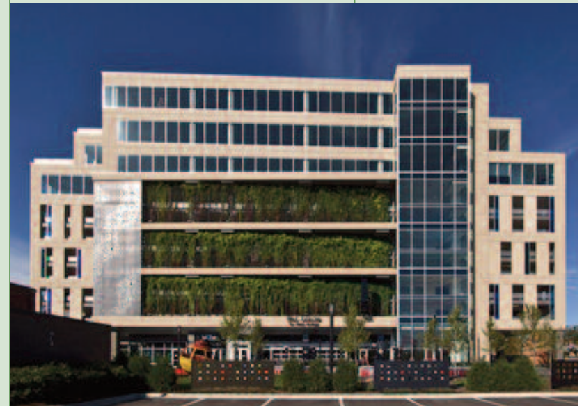
The Ackerberg Group's MoZaic building in Uptown Minneapolis is an excellent example of a vertical living green screen.
